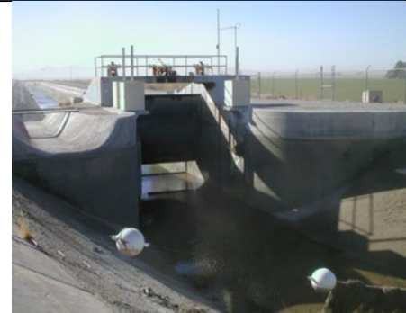
Colorado River Indian Irrigation Project, Radial Gate Structures 1 and 2 on the main canal
