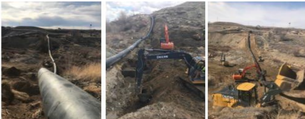
Three Bitsui Siphon Construction photos
