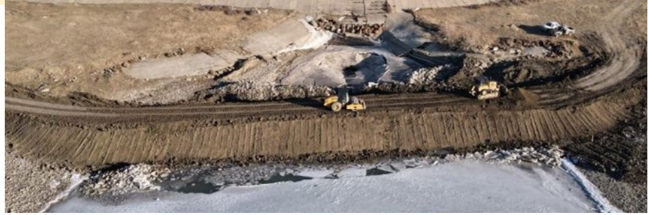
Four Horns Dam during Construction of Coffier Dam
