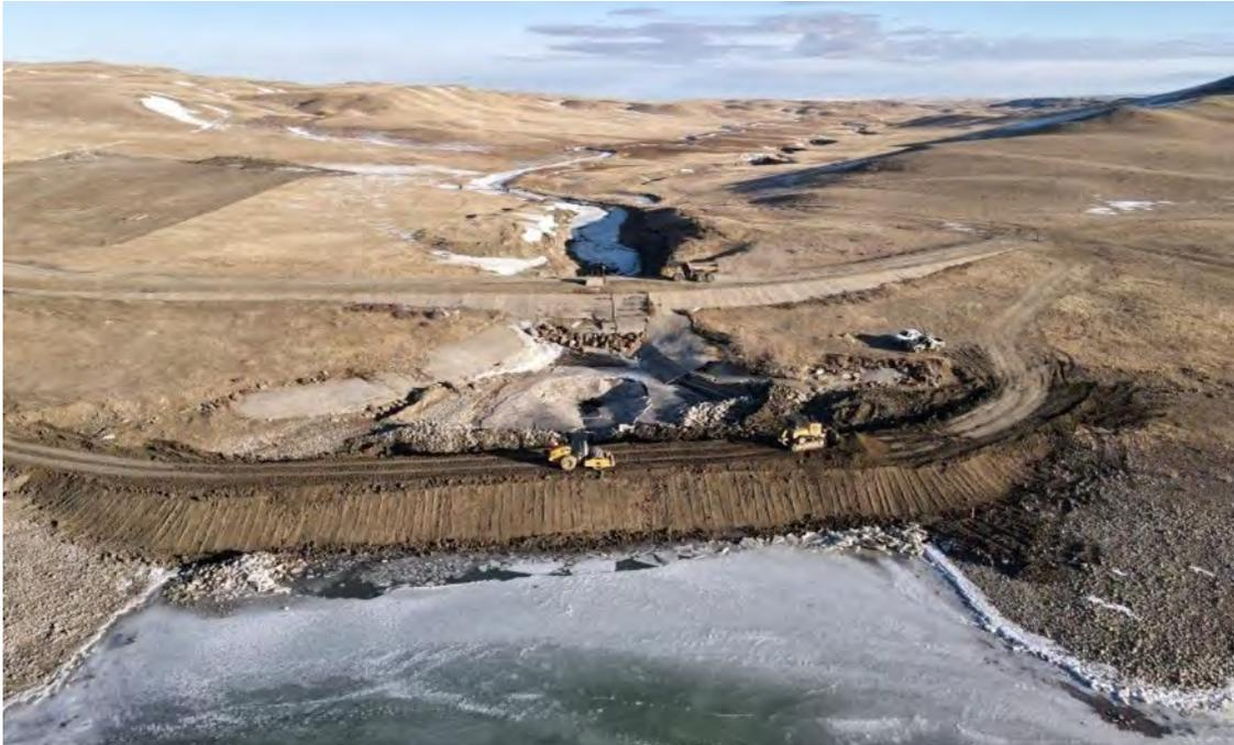
*Coffer dam in foreground, old Four Horns Dam in upper-middle of picture (November 2020)*
