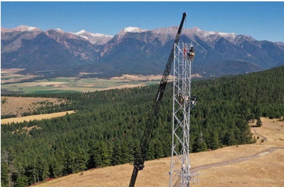
*Installation of 2.5 GHz radio frequency band tower to provide broadband services on the Flathead Reservation*
