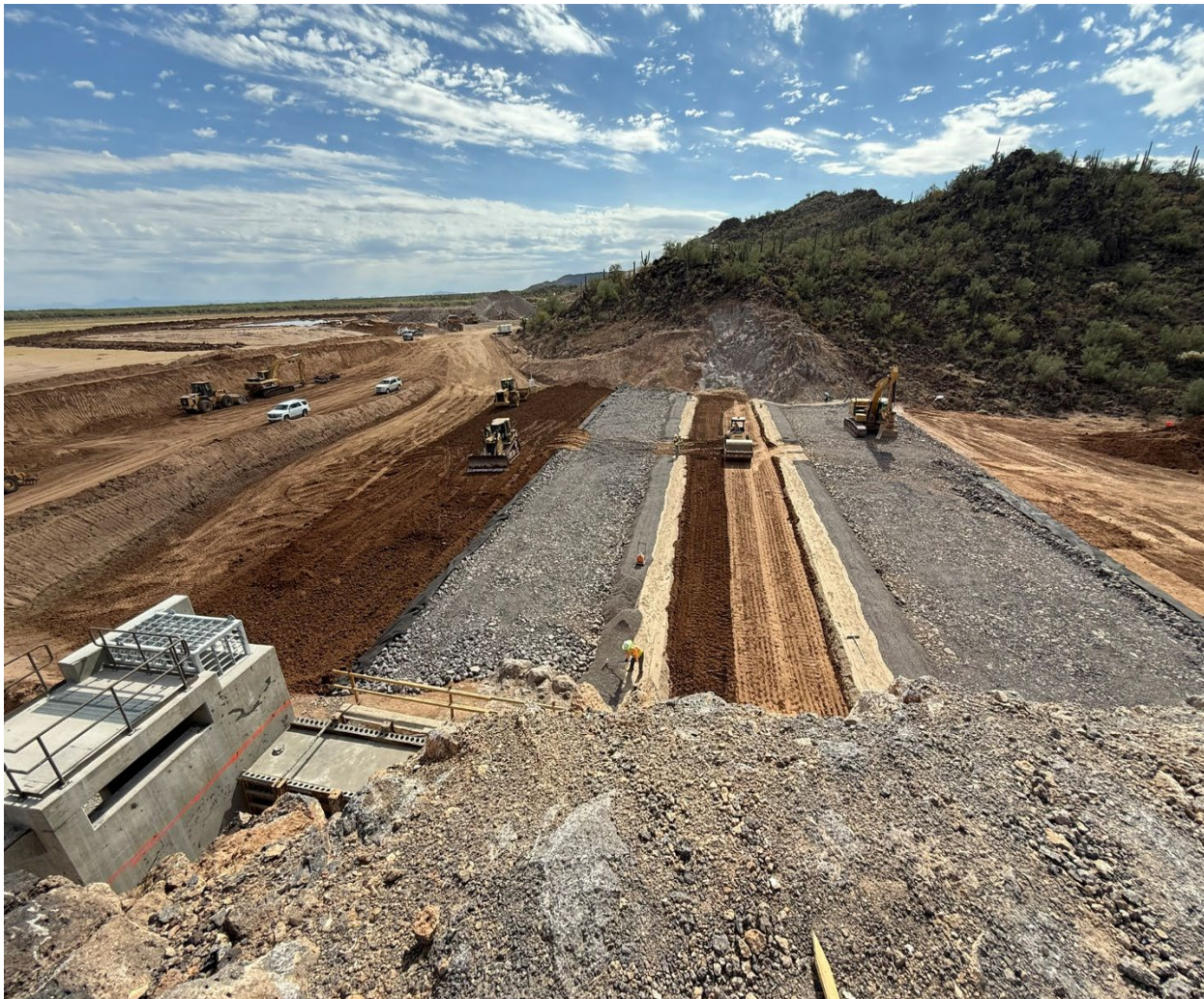
Construction of the new Menager's Dam, October 2025
