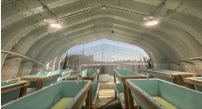
Photo shows the Aquatic Reproduction Center (ARC) water table facility, including new LED lighting, motion sensors, and circulating fans, all of which protect against the elements, reduce moisture and mold, and predation from small rodents and birds.
