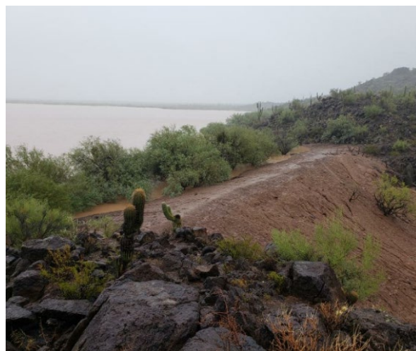
Menager's Dam during Tropical Storm Rosa, October 2018
