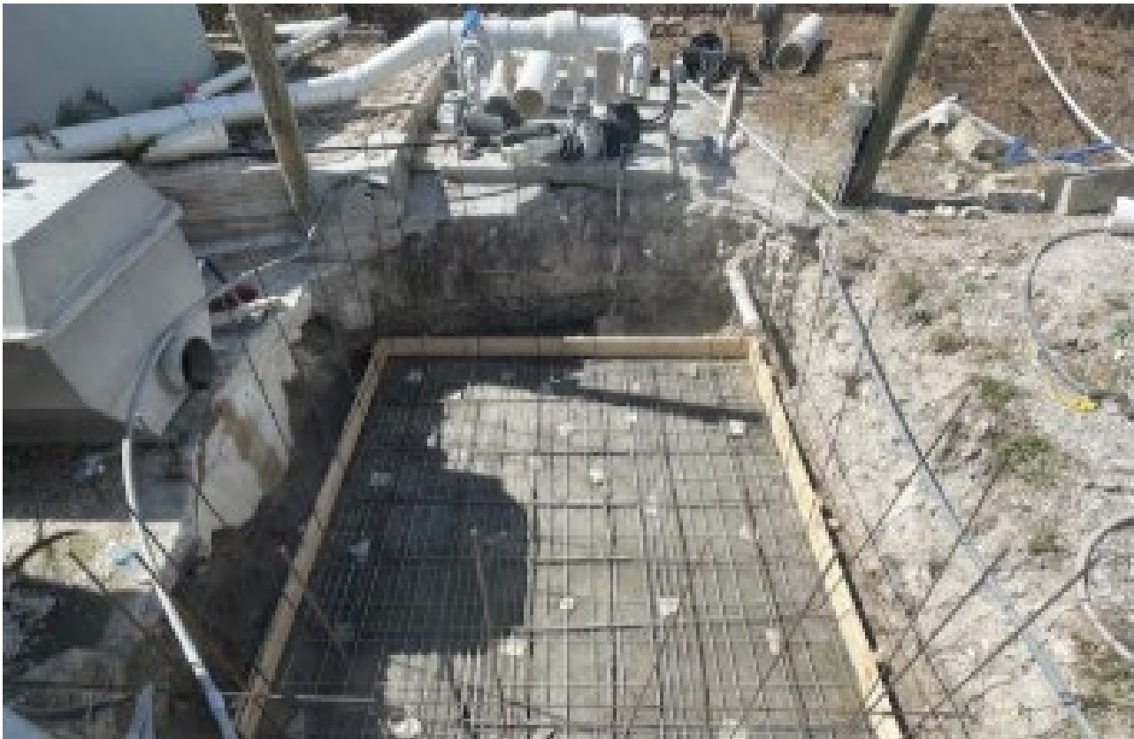
Image shows one of three sump holes being prepared for concrete and water proofing resurfacing for ARC's recirculation systems. Waterproofing the walls and floors improves durability and reduces maintenance needs.
