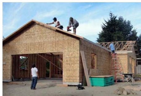
New home construction at Suquamish Tribe
