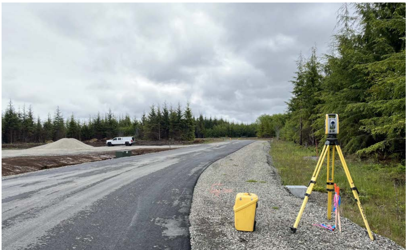
Site preparations are ongoing for construction of new homes at the Hoh Highlands, a key infrastructure project of the Hoh Tribe's relocation program
