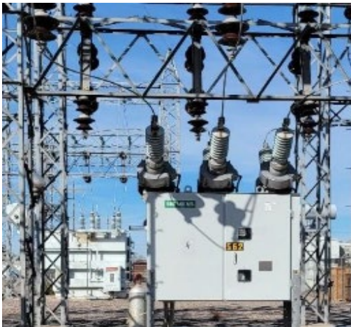
Transmission breaker at Coolidge Substation, AZ
