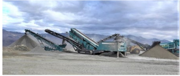
Grinding Rocks Aggregate Plant operated by the Fort Independence Tribe
