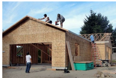
Home under construction on Suquamish Tribe reservation
