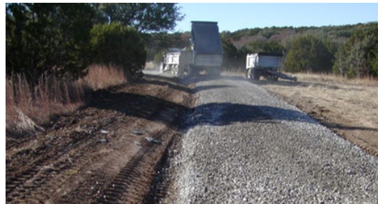
Laying down aggregate road base
