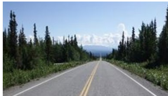
BIA transportation project completed
