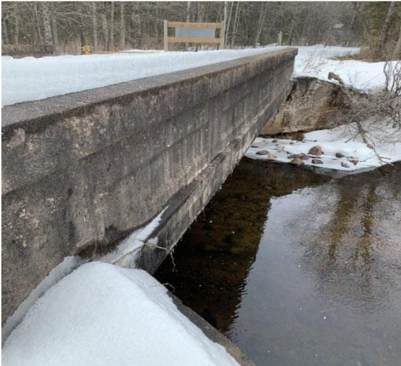
Oconto River Bridge before sampling for asbestos-containing materials.
