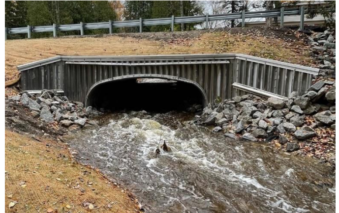
A restored culvert along Tannery Creek.
