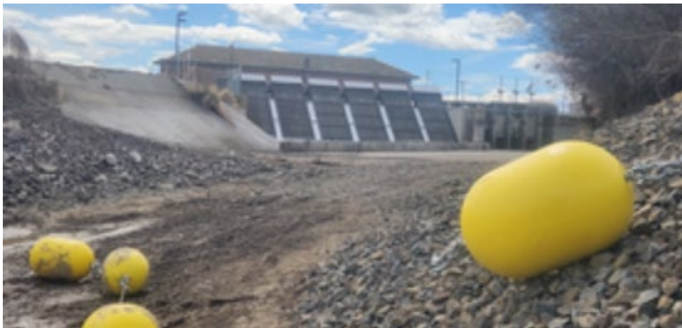
Photos of the new automated debris screening at the Drop 1 Facility (before and during irrigation delivery)
