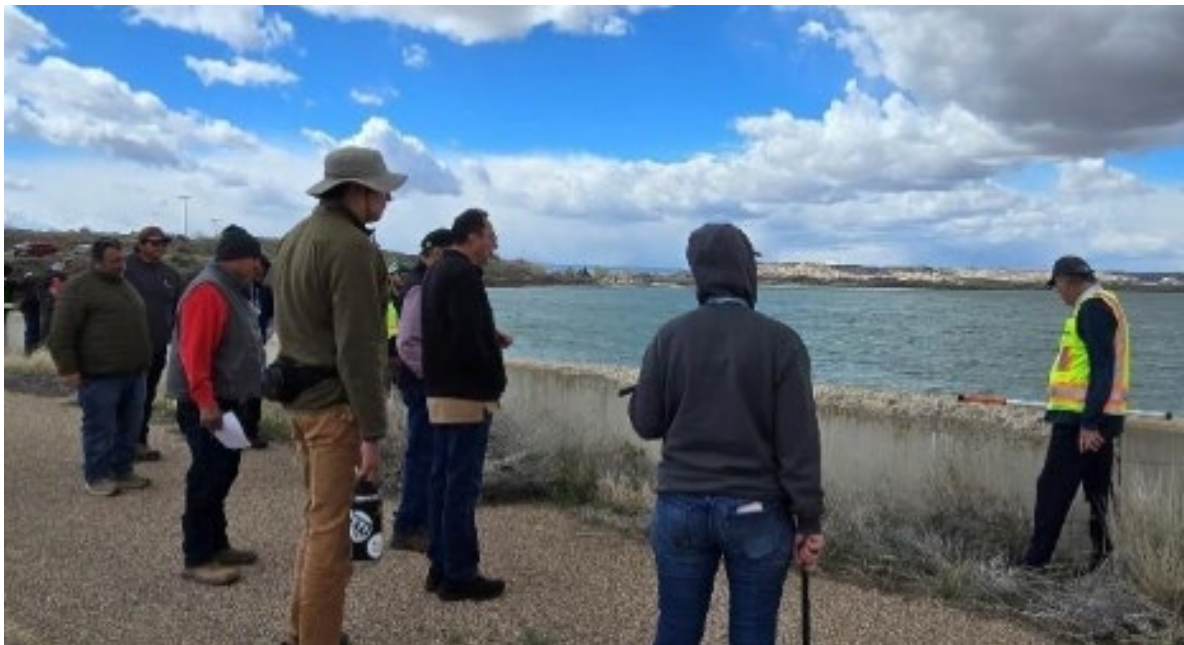
Dam Inspection at Midview Dam, Ft. Duchesne, UT
