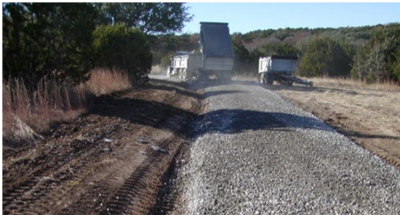
Laying down aggregate road base
