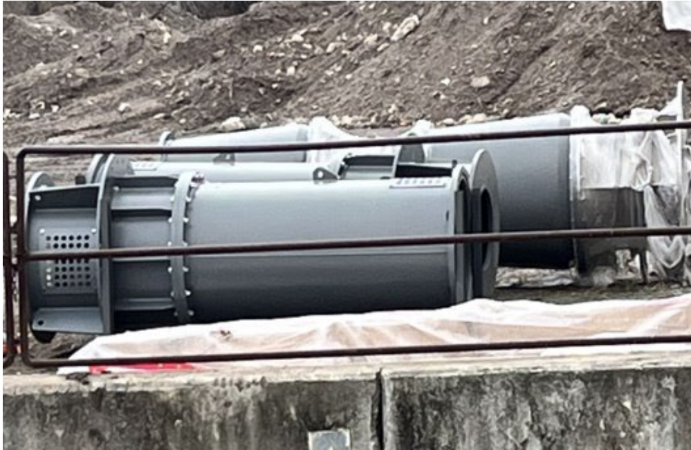
Portneuf Pumping Plant at Fort Hall Indian Irrigation Project, Idaho – new pumps ready to install.
