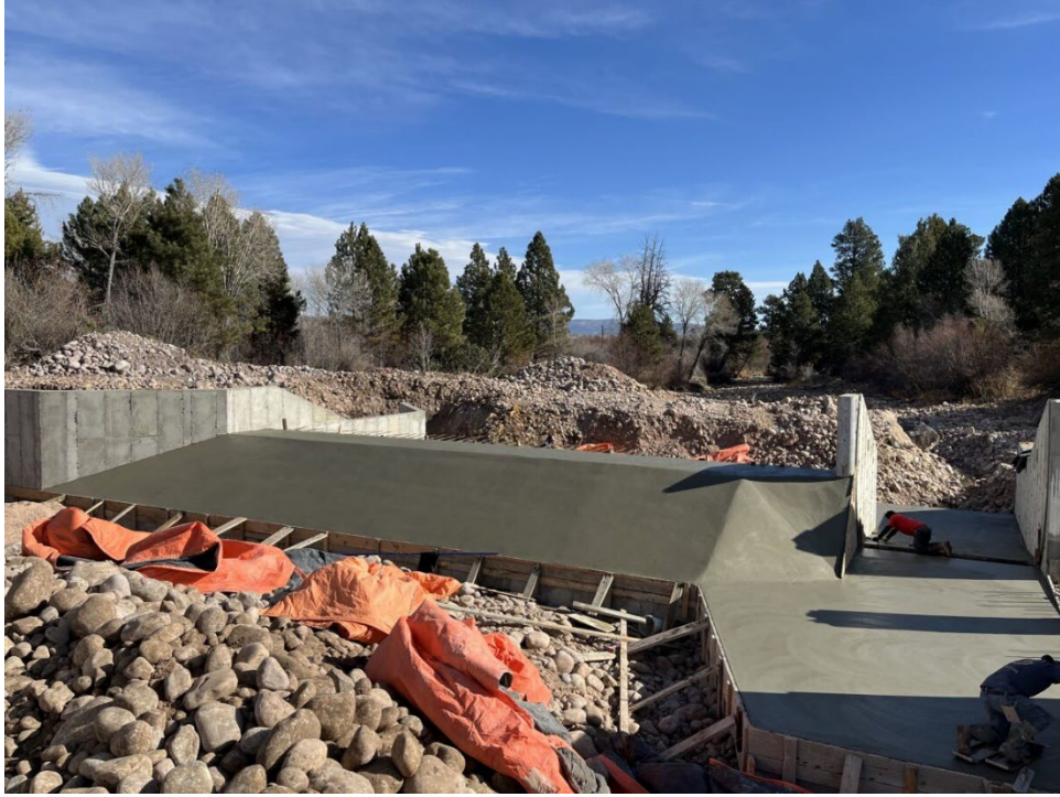
Uintah River bifurcation replacement, Uintah Indian Irrigation Project, Utah – under construction
