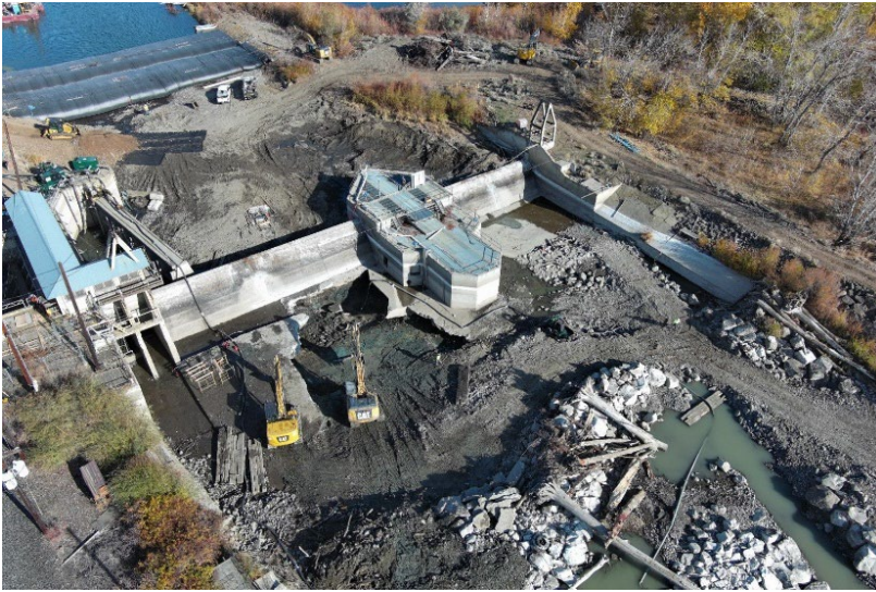
Pictured to the left: Wapato Diversion at Wapato Irrigation Project, Washington – scour hole emergency repair.
