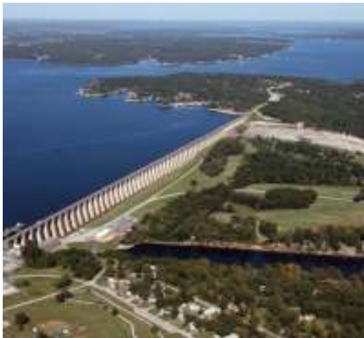
Pensacola Dam, Grand Lake O' the Cherokees
