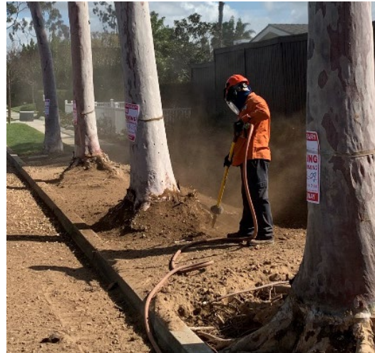
Clearing roots for assessment
