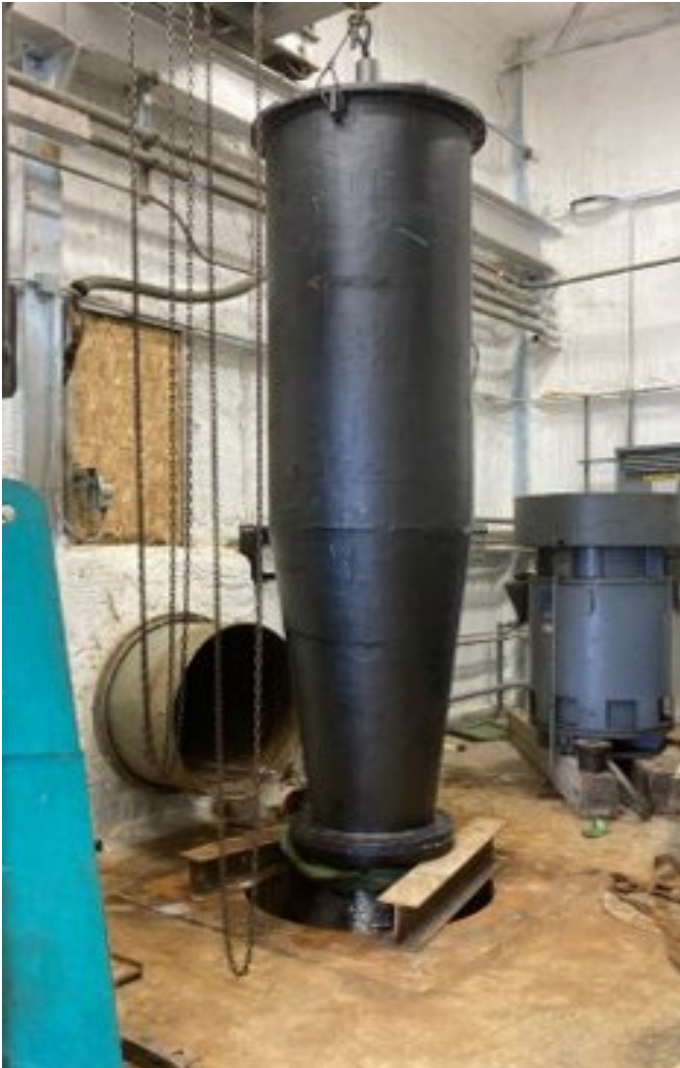
Viota Pumping Plan at Fort Peck Indian Project, Montana – reinstalling refurbished pump and housing.
