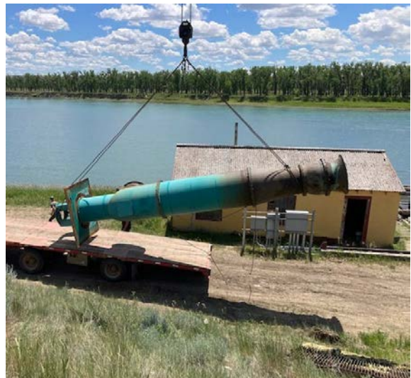
Wiota Pumping Plant at Fort Peck Indian Project, Montana – removal of old pump set for refurbishment.
