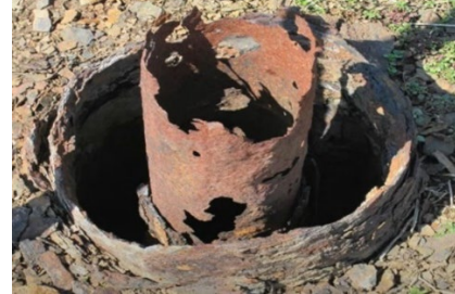
Orphan well in a field and, a well pipe visible on the ground
