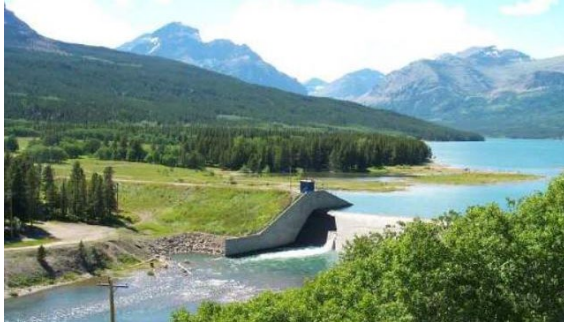
Two Medicine Dam at Blackfeet Reservation
