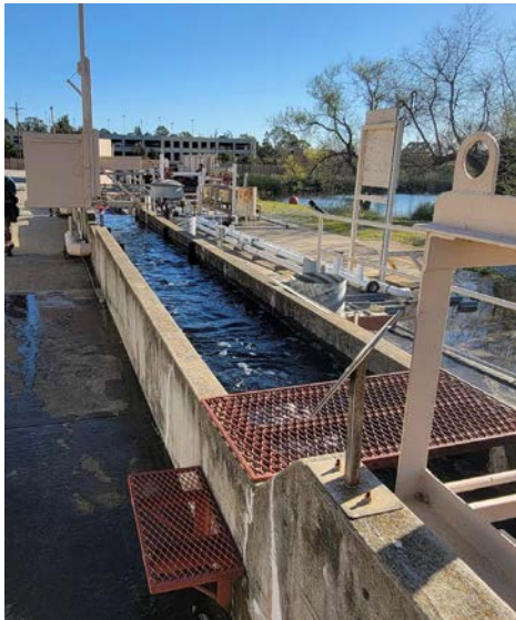
Irrigation Canal Testing at the Water Resources Technician Training Program held at California Polytechnic State University in CA
