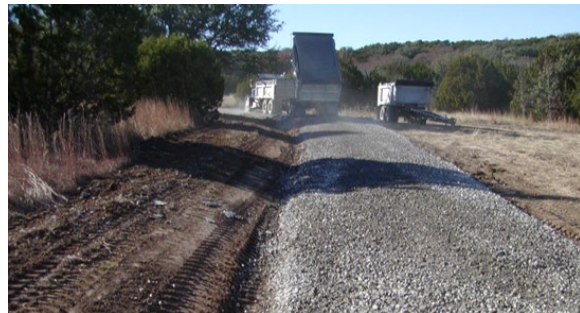
Laying down aggregate road base
