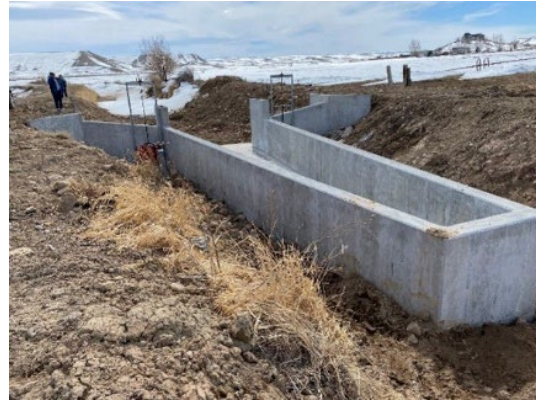
Long crested weir under construction at Uintah Indian Irrigation Project (UT)
