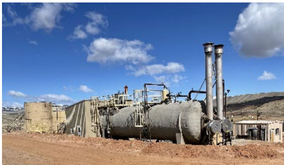
Steamboat Butte Oil Field now operating under the Tribe's Wind River Energy Commission (WREC)
