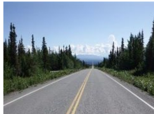
BIA transportation project completed
