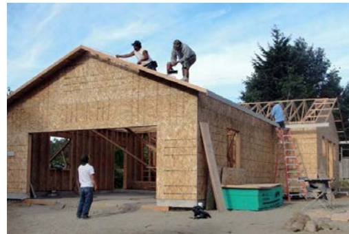
Home under construction on Suquamish Tribe reservation
