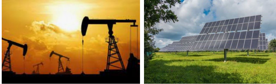
Oil rigs Wind River and solar panels on tribal land
