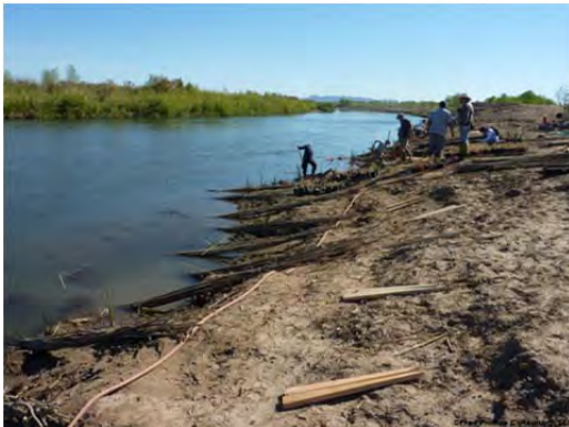
Figure 10-1. Harvested willow poles are planted along a bankline to provide additional erosion protection. Left: Work crews prep the bundles of willow poles after they have soaked in the Colorado River. Right: the same location one year after planting. Photos courtesy of Fred Phillips Consulting.
