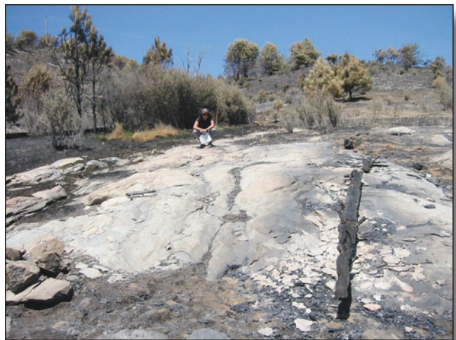
Figure 4-7 —White granitic bedrock mortar outcrop showing discoloration and spalling following a wildland fire. Spalling can be severe at rock outcrops where the fuels are heavy and allowed to radiate heat for extended lengths of time. This is graphically illustrated by the damage underneath the 24-inch dbh ponderosa pine that fell and smoldered on this bedrock mortar outcrop.
