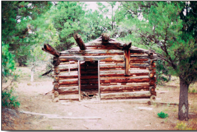
Figure 6-7—19 th century log cabin, Colorado.
