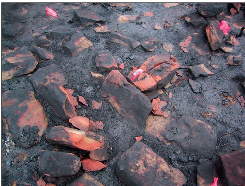
Figure 7-2 —Examples of spalling of sandstone due to heating during the 2002 Long Mesa Fire, Mesa Verde National Park, Colorado: (a) panorama, (b) close up (from Buenger 2003).
