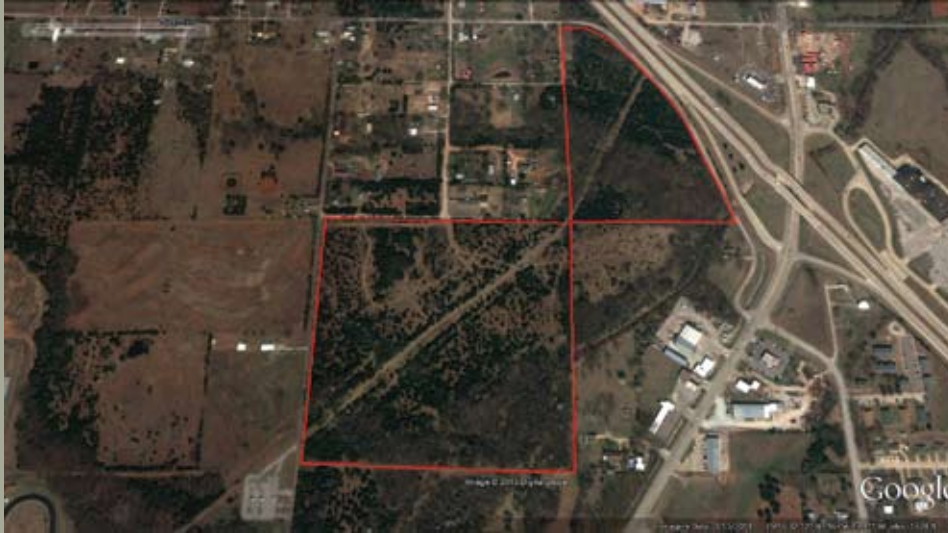
Above, pre-treatment aerial view of the project area
