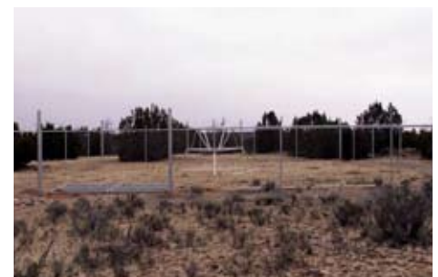
New RAWS Site under construction
