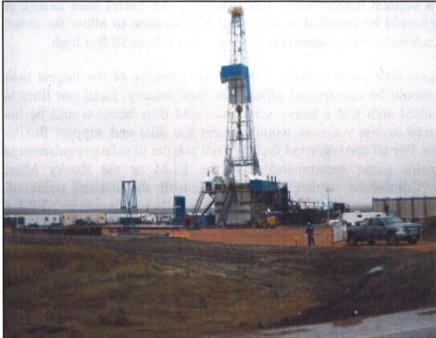
Figure 2.2. Typical drilling rig.
