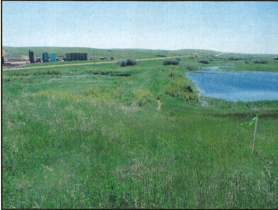
Figure 3. Photograph of Little Shell Creek Dam looking southwest along directional drill route back on Elk 16-21H pad.
