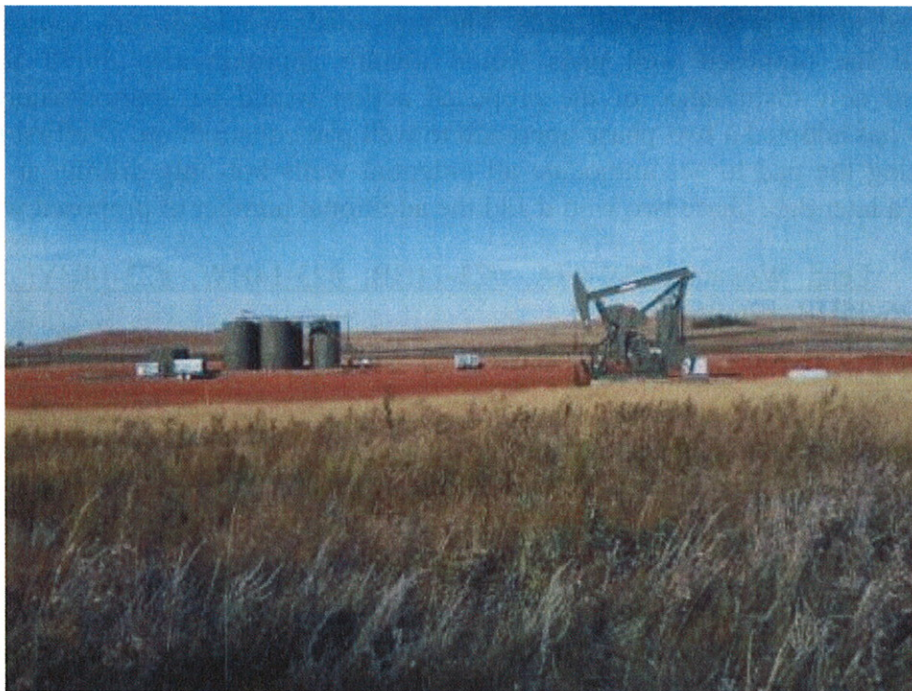
Figure 2-3. Typical producing oil well pad.
