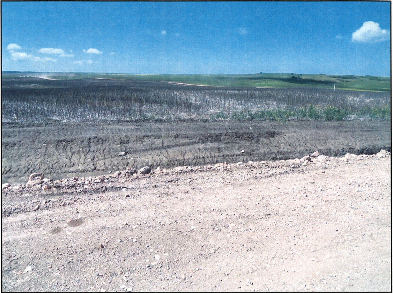
Figure 2. Proposed well pad expansion area photograph.
