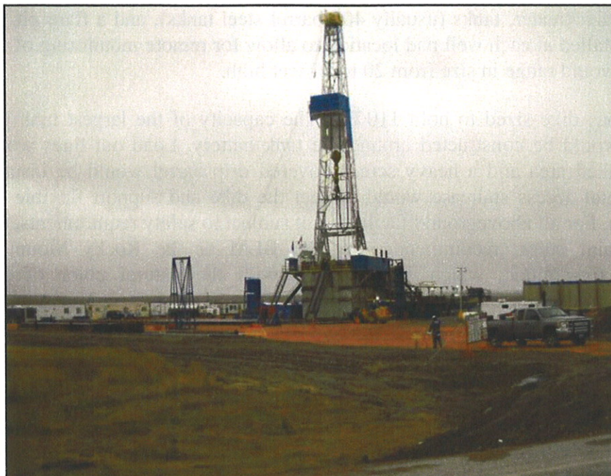
Figure 2.2. Typical drilling rig.
