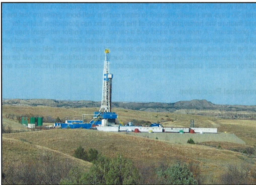
Figure 4. Typical drill rig (Carlson McCain)
