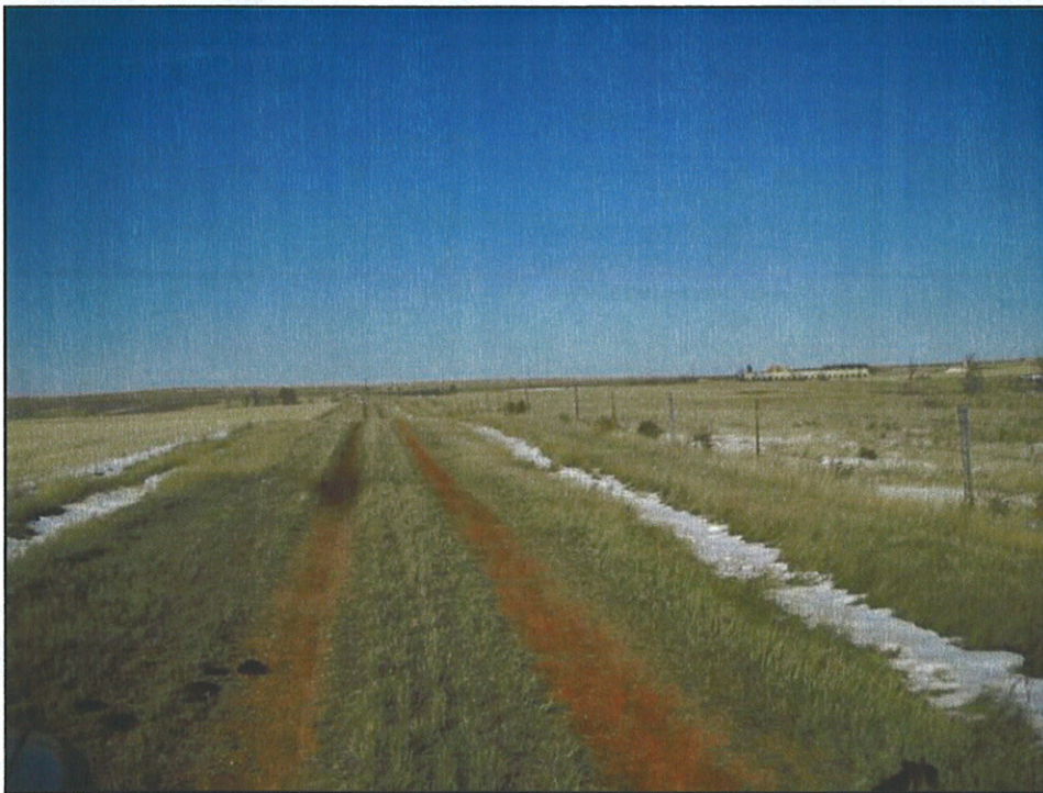
Figure 14. Riverview Section 31 access road area, facing south.
