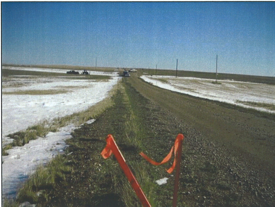
Figure 8. Hawkeye Section 24 access road area, facing east.
