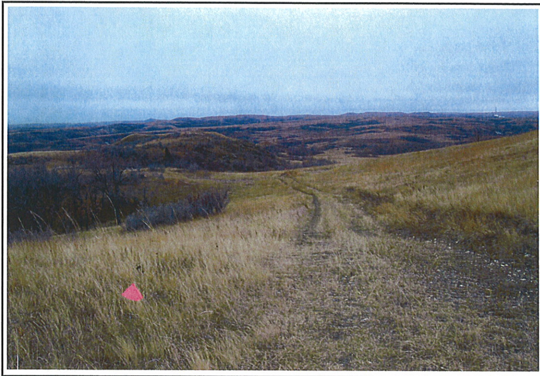
Photograph # 3 Date: November 15, 2010 Direction: South Subject: Proposed new access road.
