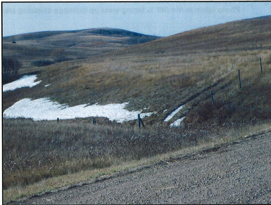
Figure 6. BIA 612 and drainage crossing. Boring will be utilized to cross SW under road and drainage.
