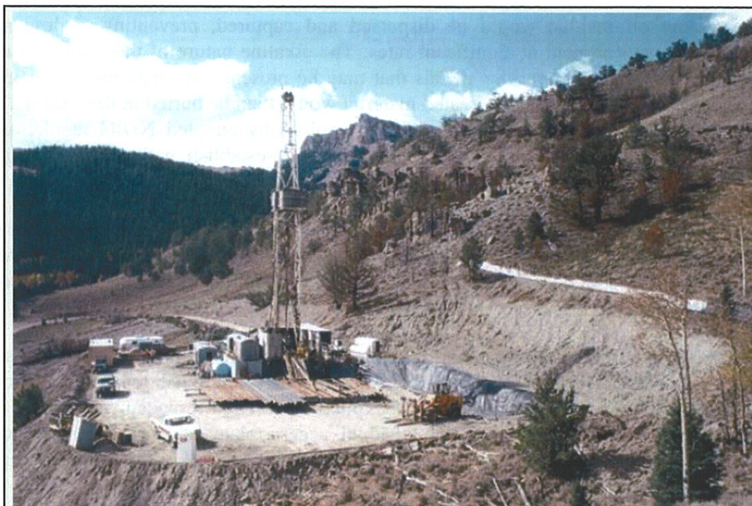
The well pad and access road are constructed to the minimum size necessary to safely conduct drilling and completion operations.
