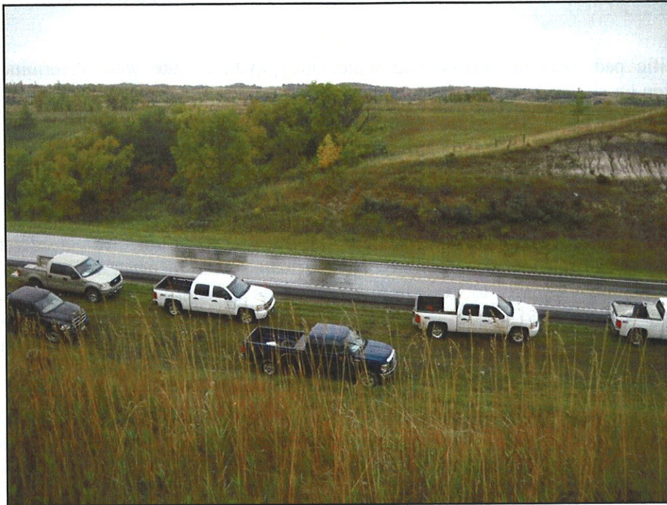
Figure 2. Bear Den #18-21H access road, facing west toward Highway 22.
