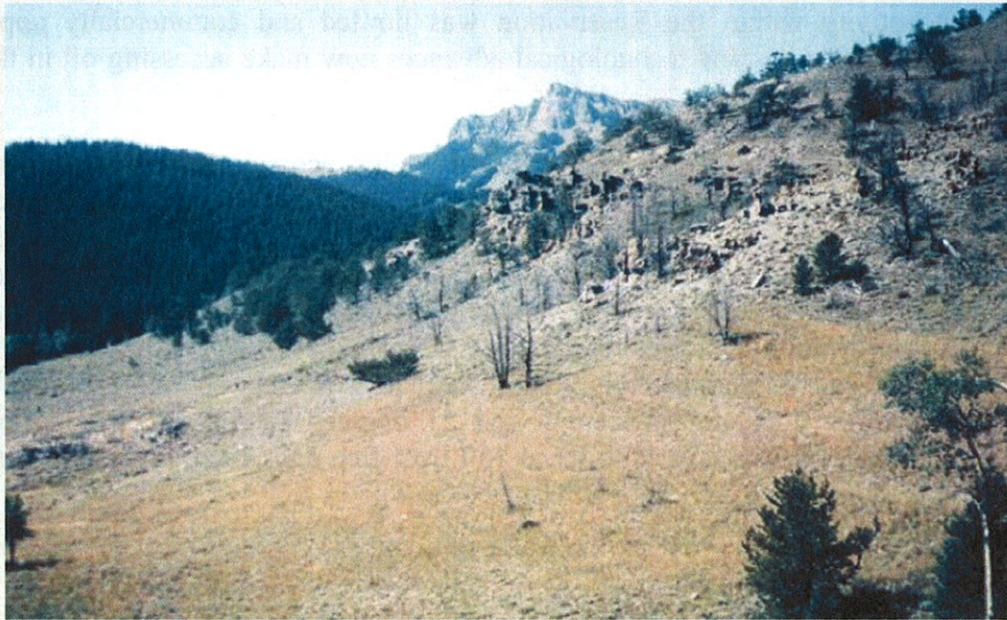
The well pad and access road have been recontoured back to the original contour, the topsoil respread, and the site revegetated.
