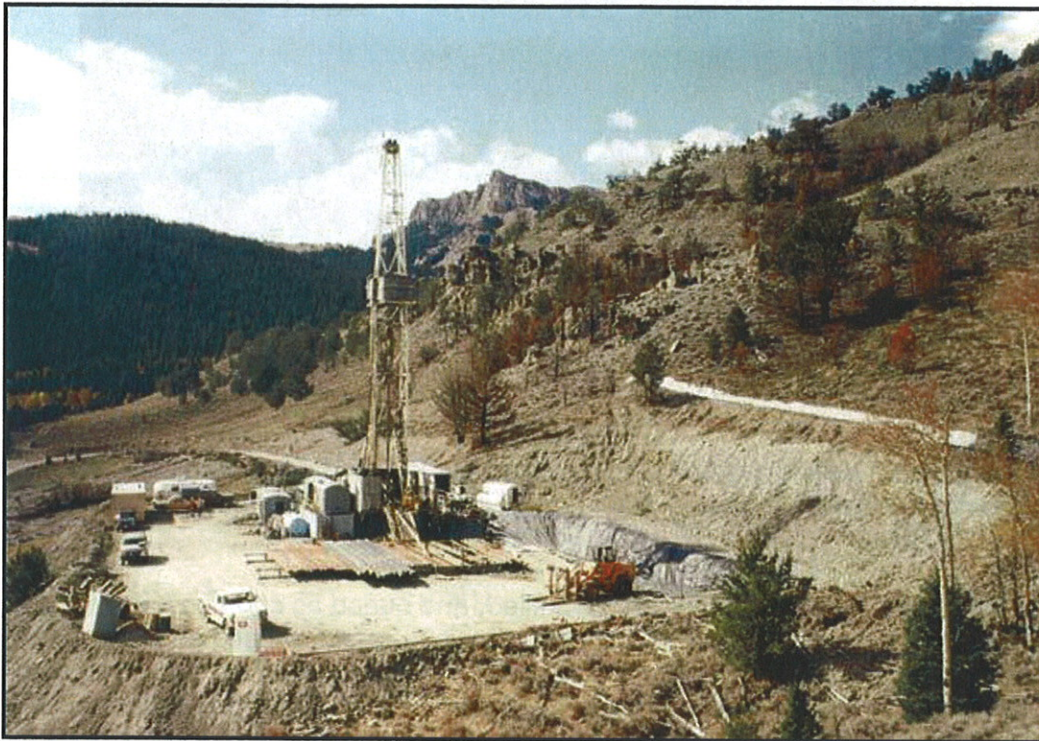
Figure 13. Typical well pad during operation.
