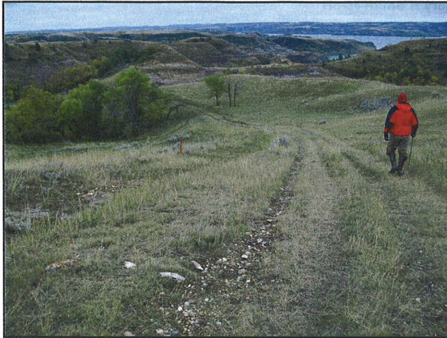
Figure 7. D-3 Hidatsa #23-26H Access Road.
