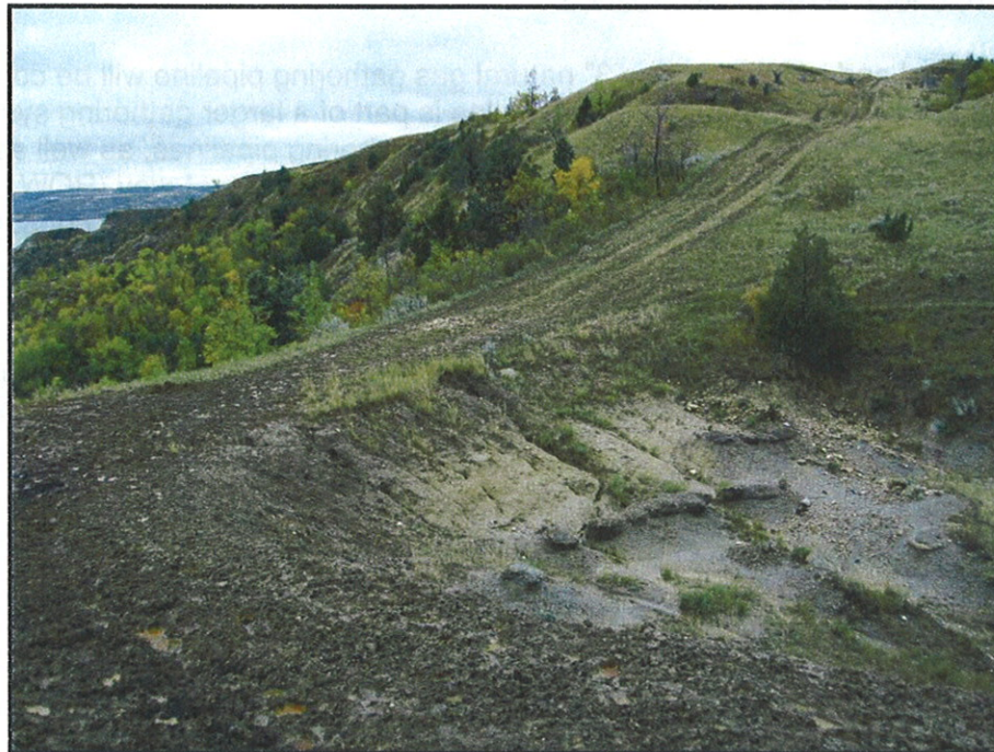
Figure 8. D-3 Hidatsa #23-26H access road ridgeline crossing.
