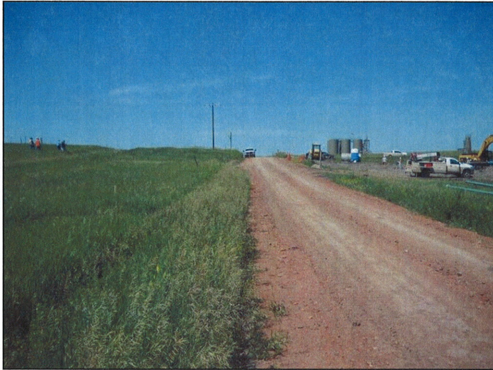
Figure 8. Horse Camp #03-16H access road, facing west.
