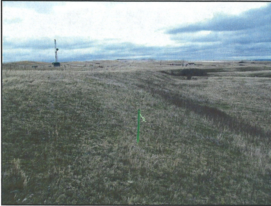
Figure 8. Route staked on side-slope in Section 16.
