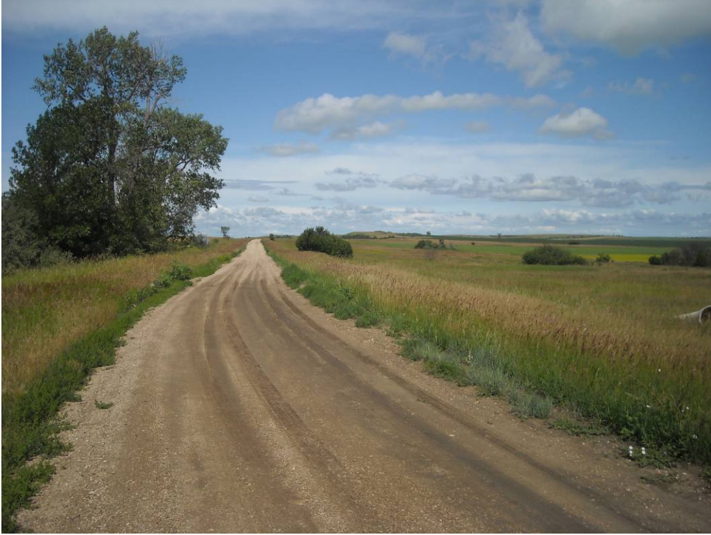
Figure 2.2a. Proposed upgraded and improved access road (BIA 5) for the Eagle 14-30H well pad, facing west.
