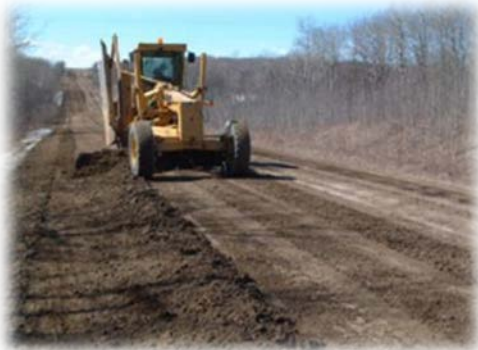
Road under construction
