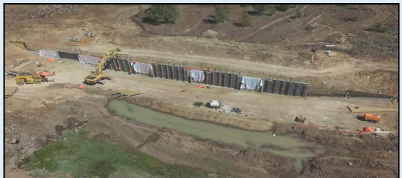
Forming the Lauer Dam's Core Wall
