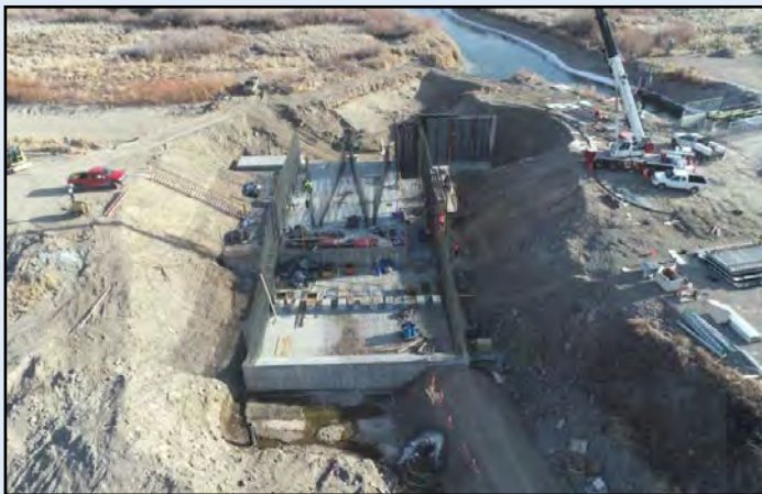
Equalizer Dam Labyrinth Spillway under construction
