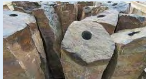
6-inch holes drilled in basalt rock
