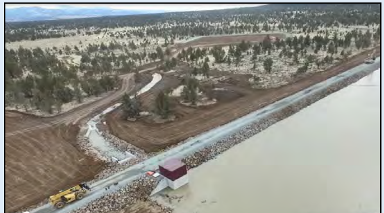
New Lauer Dam during first filling
