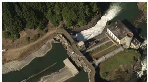
Elwah Dam prior to demolition
