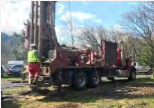
View of air rotary drill rig used to install the replacement water well
