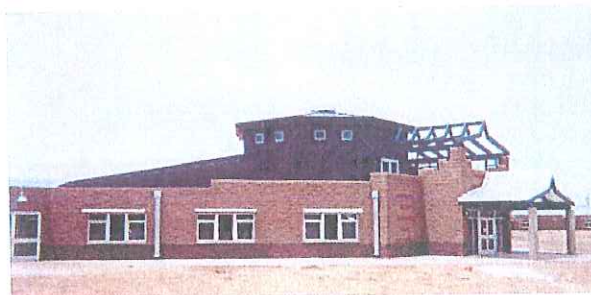
Seba Dalkai Boarding School, Arizona OIG Photo
