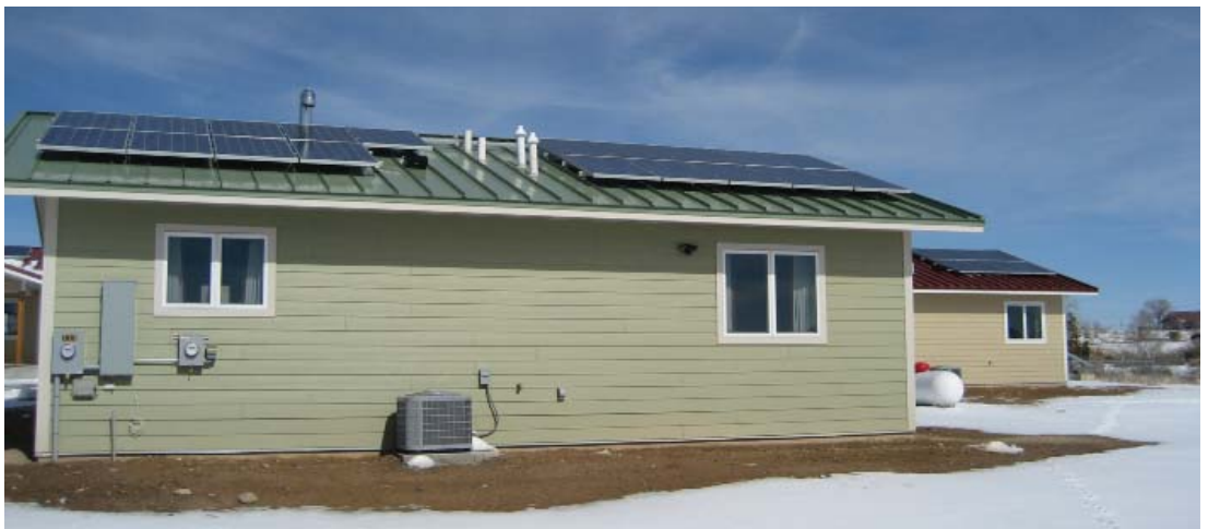
Above: Rooftop solar electricity panels lead to this converter box (right).
