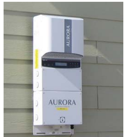
Above: Rooftop solar electricity panels lead to this converter box (right).
