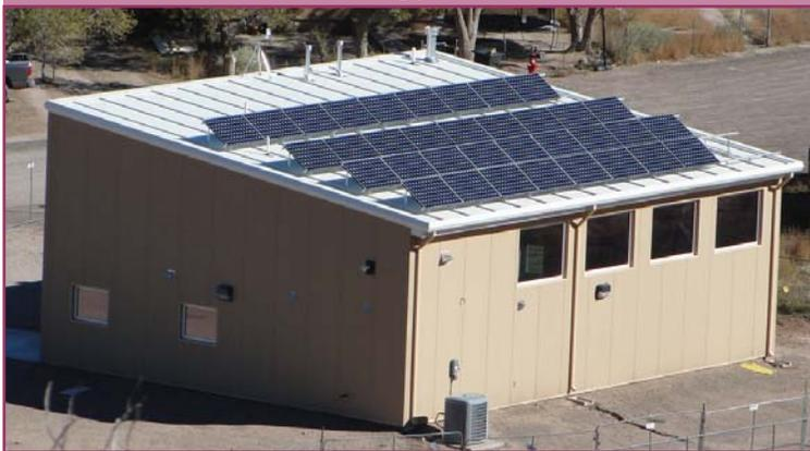
*The 1,980 square foot Nazlini Community School Fire Station opened in May. It will produce at least 75 percent of its required energy using roof-mounted solar photovoltaic panels which generate approximately 9.9 kW.*
