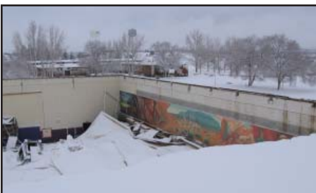
The gym at the Shonto Preparatory School in Arizona is being repaired following a 2010 roof collapse.
