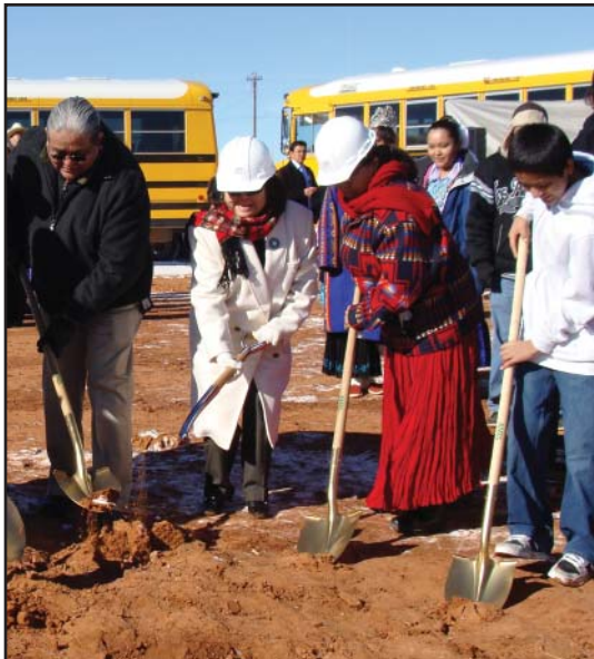
From left: OFMC Deputy Director Emerson Eskeets, School Board Members Darnell June and Marie Martin and 8th grader Brandon Benally participate in the January Kaibeto Boarding School groundbreaking.
