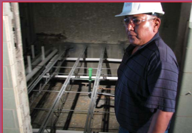
Sherman Indian High School Facility Manager Leroy Tewahaftewa views a gutted shower room in a dormitory at the California school.
