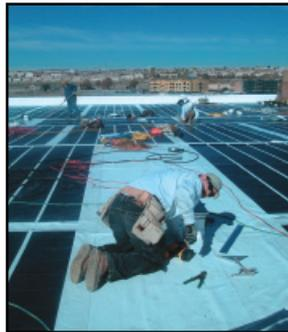
The solar photovoltaic membrane was installed on SIPI's gym roof in 2008.
