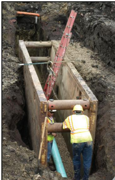
Workers utilize a trench box to guard against cave-ins during their water and sewer pipe installation.
