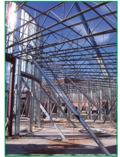
Constructing Baca / Dlo'ay Azhi Community School, a LEED Certified BIA school.
