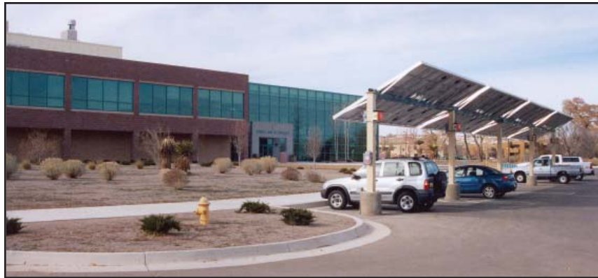
Solar panels in the SIPI Science and Technology Building parking lot track the sun
