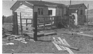
Blackfeet – Renovation (before)
