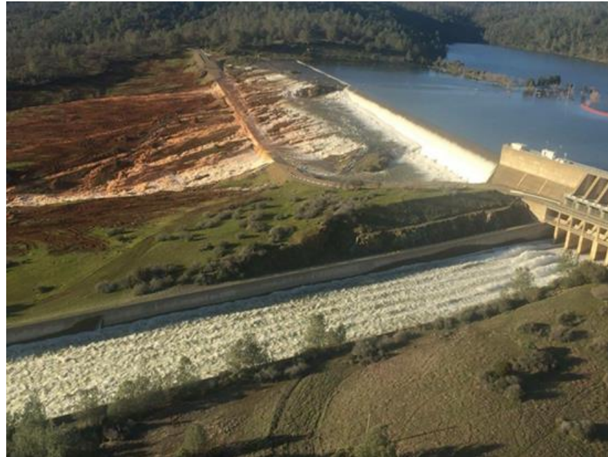
(Picture from news helicopter, showing water flowing over the emergency spill way)
