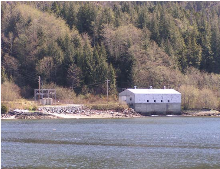
Figure 16: Purple Lake Hydroelectric Plant
