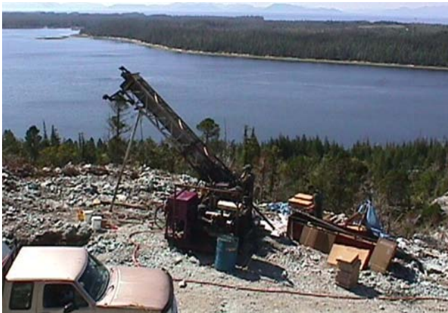
Figure 5: Core Drill at Bald Ridge Site
