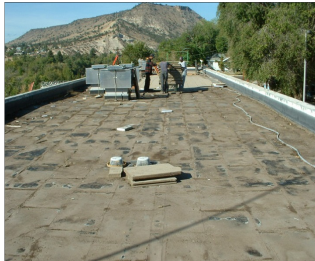
A roof is being repaired at the Warm Springs Detention Center, OR.
