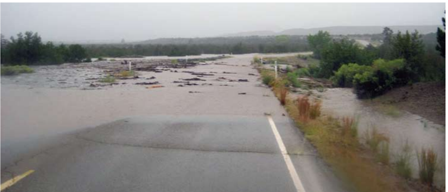
Cochiti Hwy-Bland Canyon road crossing on September 13, 2013.
