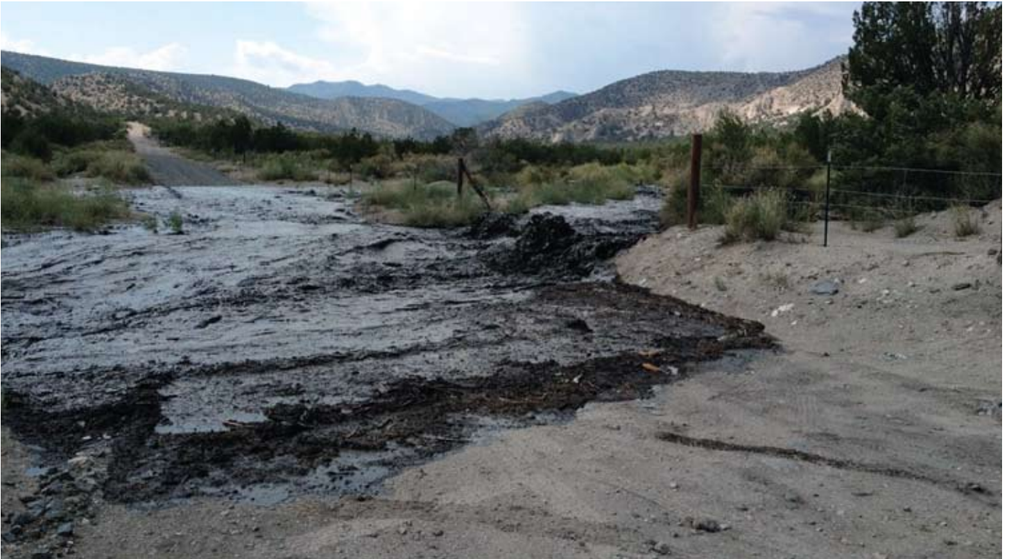
Peralta Canyon low-water crossing.
