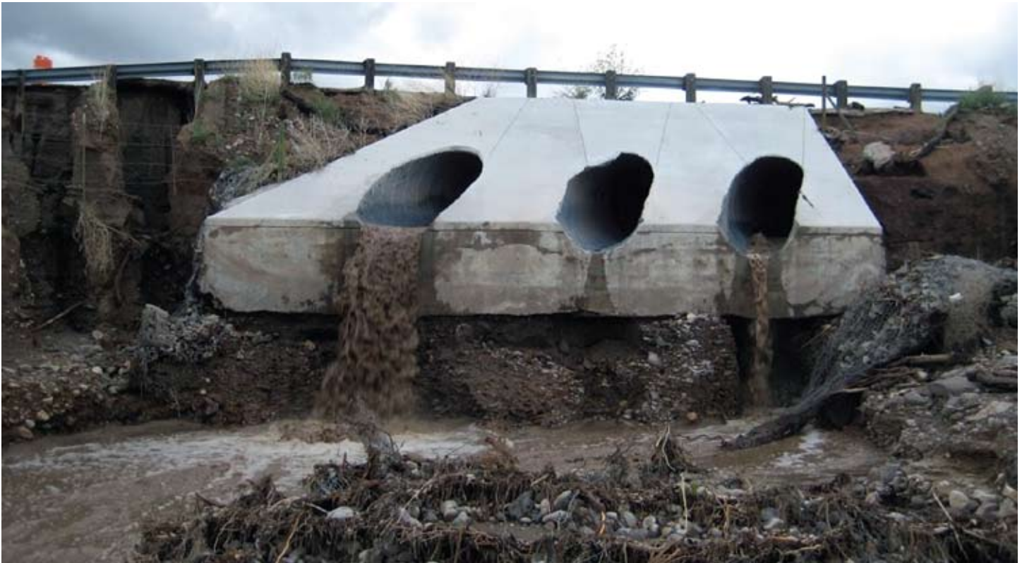
Cochiti Hwy-Bland Canyon road crossing - downstream of culvert crossing.
