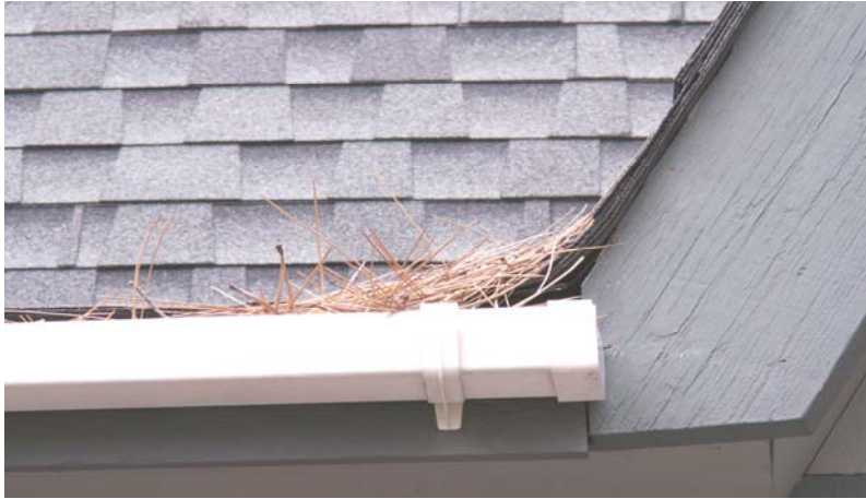
Gutters should be kept clean.
